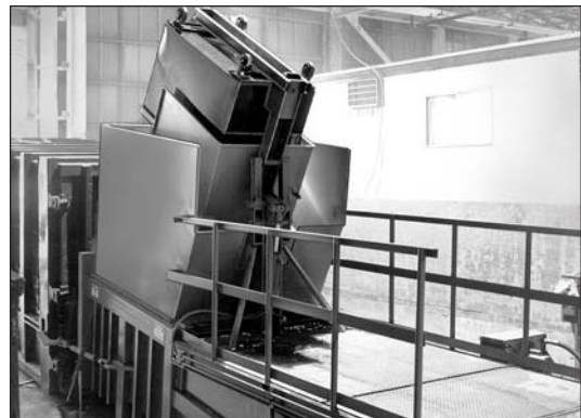
Deck Dumper Installation
