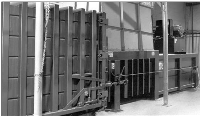
Transfer Station Installation
